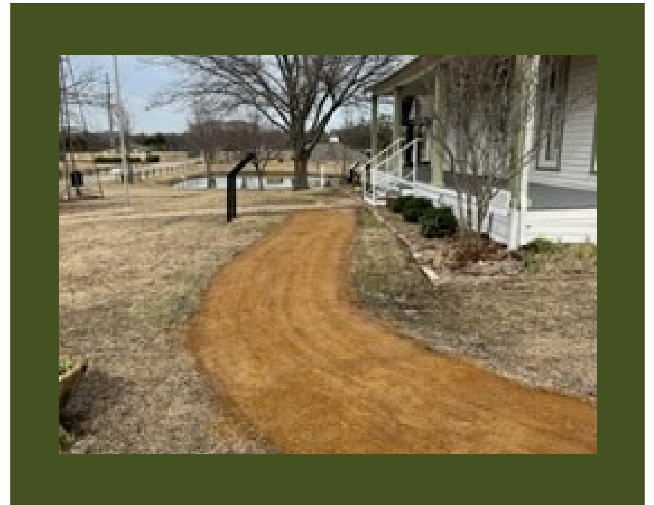
ROCKWALL MUSEUM GRANITE TRAIL INSTALLATION
